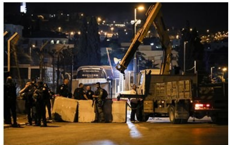
Israel forces place cement blocks at the entrance of Sheikh Jarrah neighbourhood of East Jerusalem Photo Credit: Ammar Awad /
